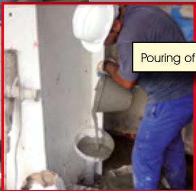
Sealing of the drilled holes for the air vent while the mortar is poured.
